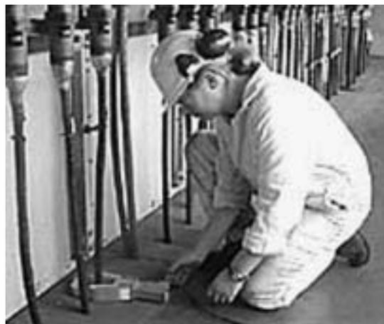
Figure 3. Clip-on CT Around Supply Cable.
